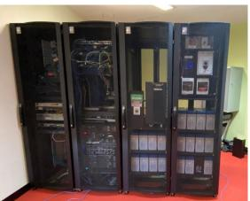
Inverters and batteries replacing the 8 year old UPS to give better energy security as well as lower energy costs.
